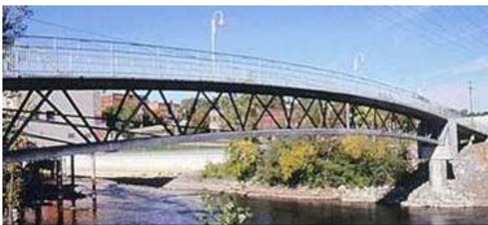
Figura 1-4 –Sherbrook Footbridge, Canada (1997). Luce: 60 m, resistenza a compressione: 200 MPa
